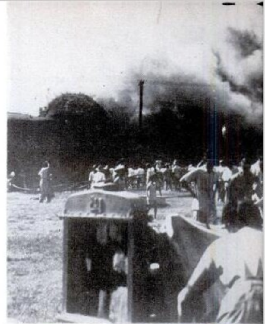
A NEWSPAPER BUILDING WITHIN MANILA'S WALLED CITY
