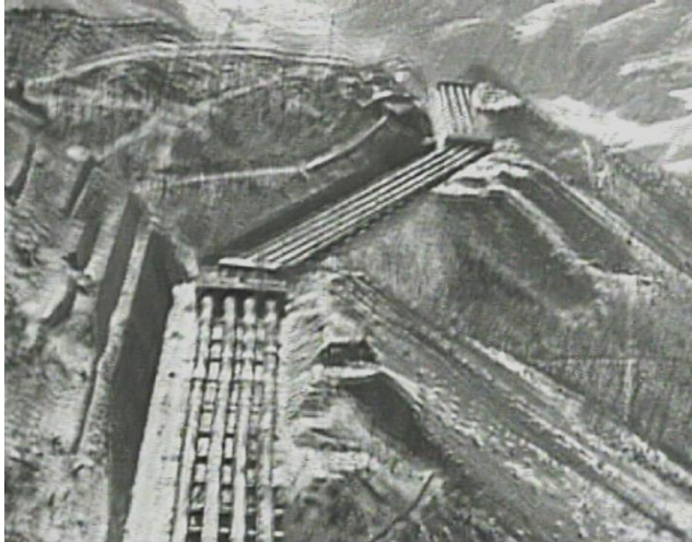
The penstocks extending south to Changjin Hydroelectric Power Plant Number 1 near the Funchilin Pass. November, 1950
