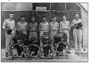
16<sup>th</sup> Photo Lab Technicians with the Aerial Cameras used on the F-13. Note the K-20 Camera Held by the Man on the Far Right – Source: U.S. Army
