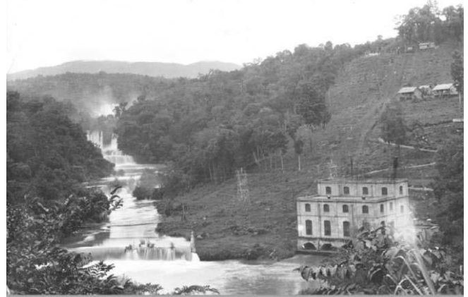
Mansam Falls and Power Station: One of three hydro-electric and one diesel power stations owned by the Burma Corporation.
