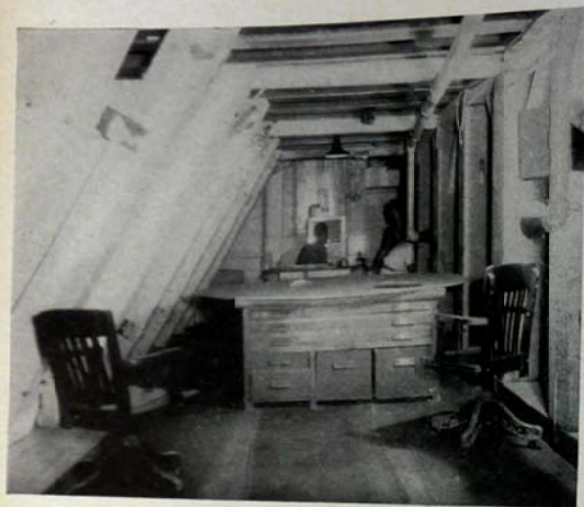
PHOTO 29 Inside main room in base of Admiral's Command Post showing central switchboard, operations table, and speaking tubes. Note heavy timber construction.
