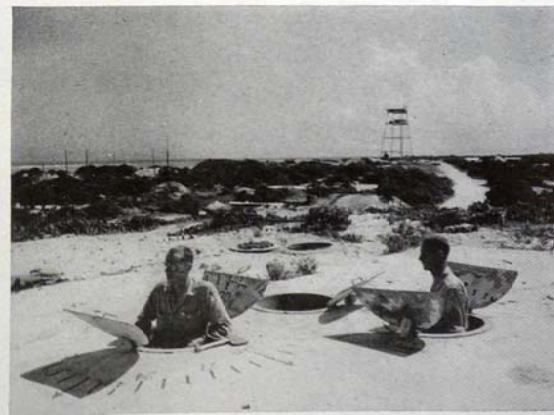
PHOTO 28 Observation hatches on top of Admiral's Com- mand Post. From this vantage point the ad- miral directed the defenses of the island com- municating with the central switchboard below by means of speaking tubes.
