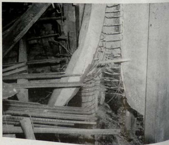
PHOTO 34 Interior of power plant showing damage caused by naval shell. Note broken steel wall column.
