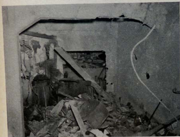
PHOTO 49 Interior of command post and fire control center showing effects of hits by naval shells during raid of July 1945. (Ref. Annex B, Section 2, Map 1, Point 18.)
