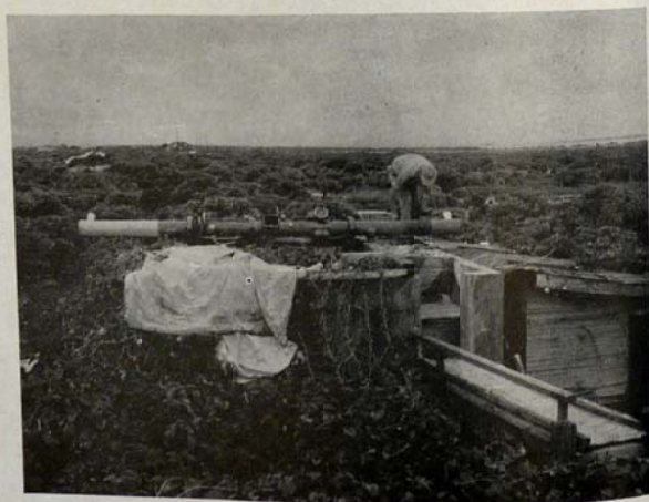
PHOTO 50 Optical range finder emplaced on top of command post and fire control center, shown in Photo 49.
