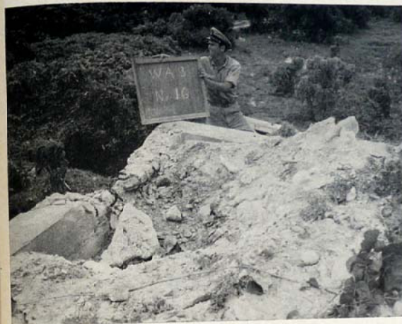
PHOTO 49 Interior of command post and fire control center showing effects of hits by naval shells during raid of July 1945. (Ref. Annex B, Section 2, Map 1, Point 18.)
