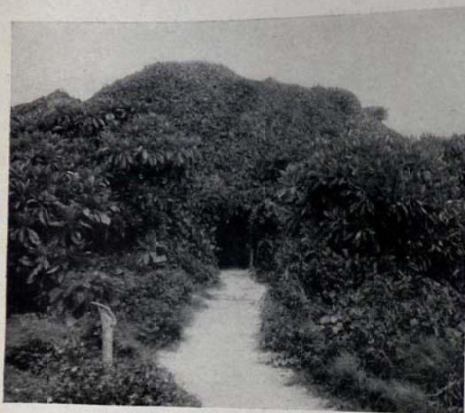
PHOTO 81 Entrance to underground surgery. Structure was made of reinforced concrete and covered with 15 feet of coral. (Ref. Annex B, Section 2, Map 4, Point 5.)
