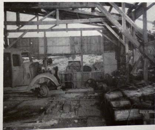
PHOTO 72 Damage to garage caused by bomb blast from near miss, probably from instantaneous fuzed 500 or 1,000-pound bomb.
