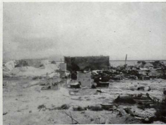
PHOTO 32 Main power plant. To the left are 2 fuel tanks of U. S. construction. In the foreground is a completely destroyed kitchen area. Notice the shell hole in power plant. Looking south.
