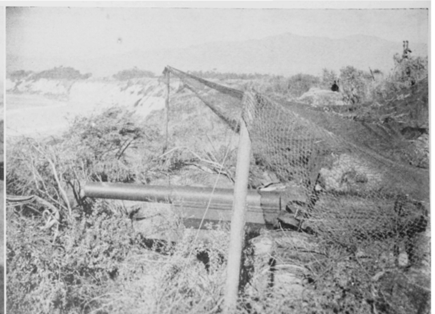
Another emplacement near Santa Barbara
