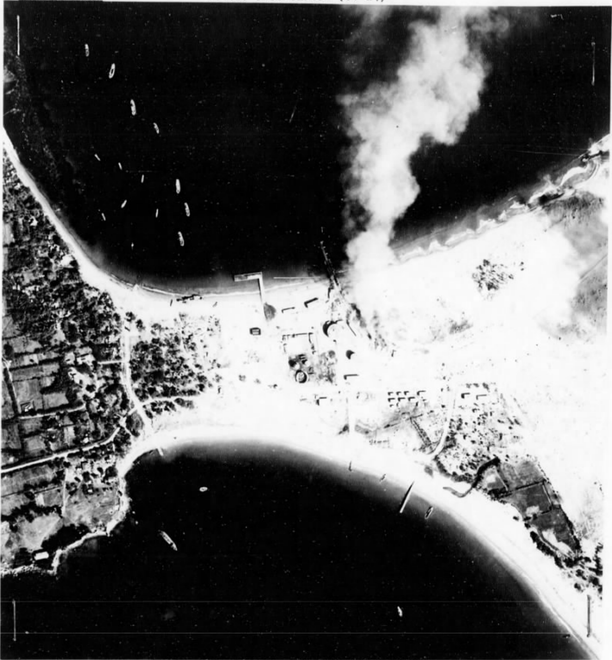
PORO OIL STORAGE, SAN FERNANDO HARBOR
