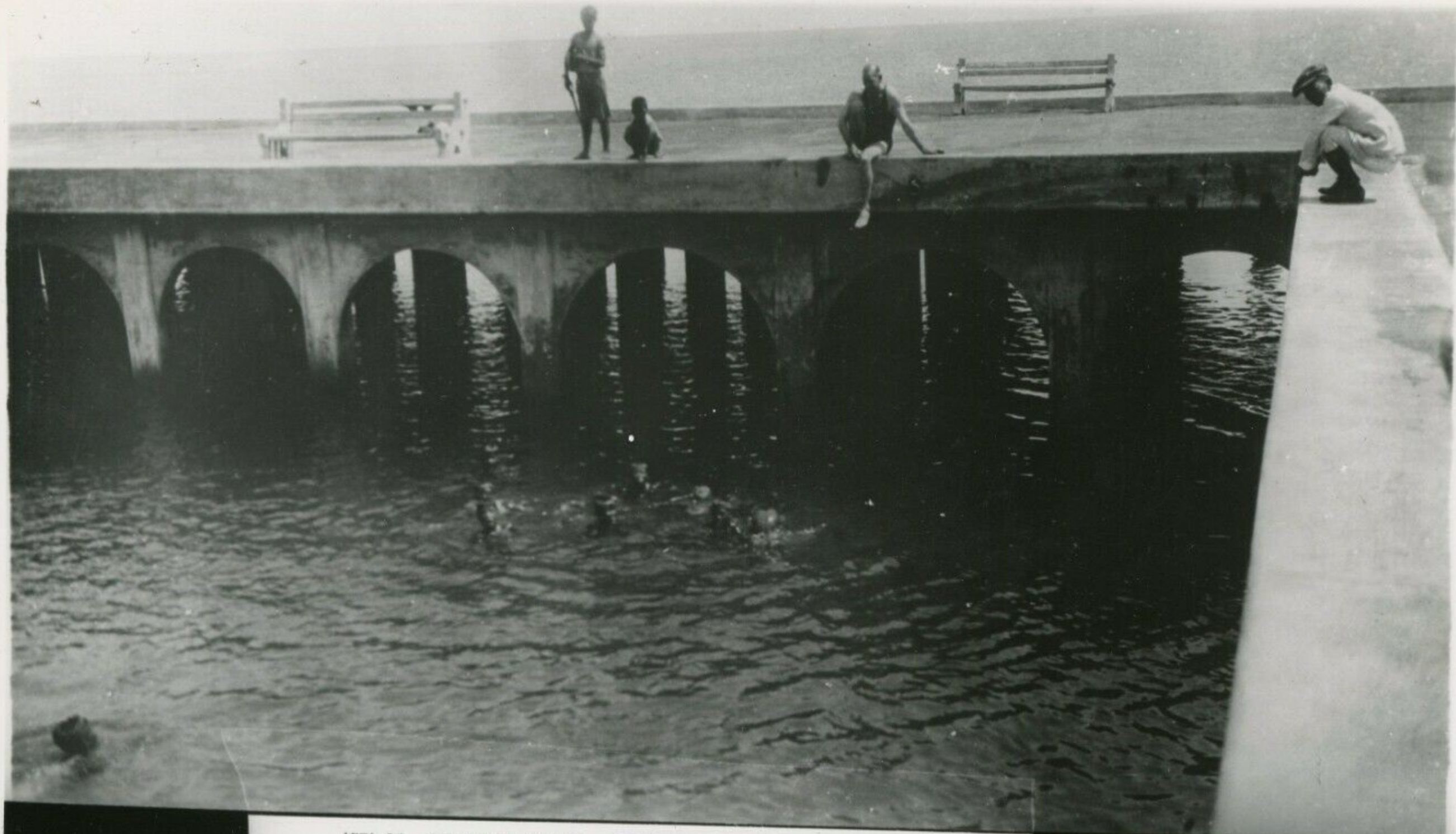
AREA 18. PHILIPPINE ISLANDS - LUZON ISLAND - LA UNION PROV. - PORO. App. Lat. 16° 34' N. - Long. 120° 17' E. The more westerly of Poroc's two piers. 1938. Encl3S-6. ONI (P-5) #351-158.
